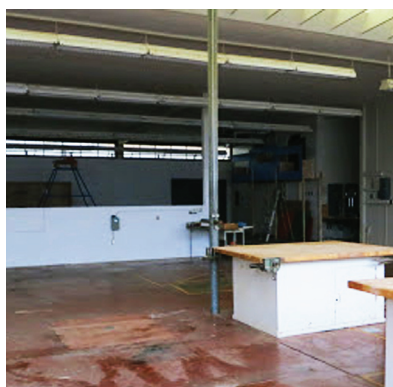
After many long hours of cleaning, the space is finally ready for the field to be completely set up.
